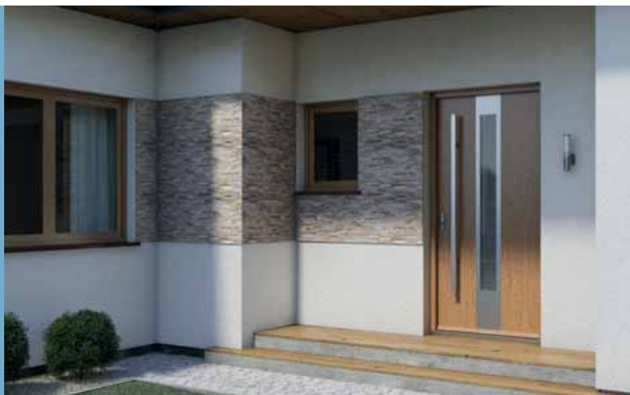
Steel SAFE E.1, Dąb Winchester
