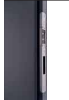
Electric strike to support the primary lock
