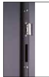
Electric strike for use with the main lock Metal door frame
